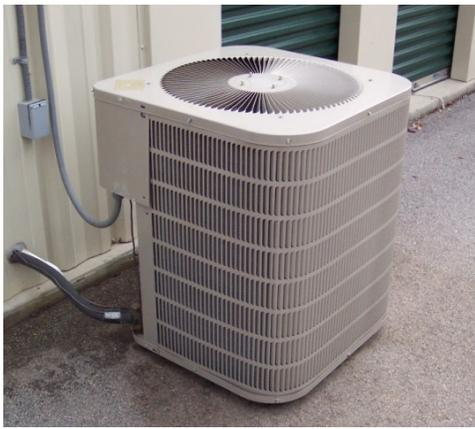
units for one interior area, set one at a lower temperature than the other. This is equivalent to undersizing the unit, a common technique for climate-controlled storage developers using conventional HVAC systems without dehumidifiers.
